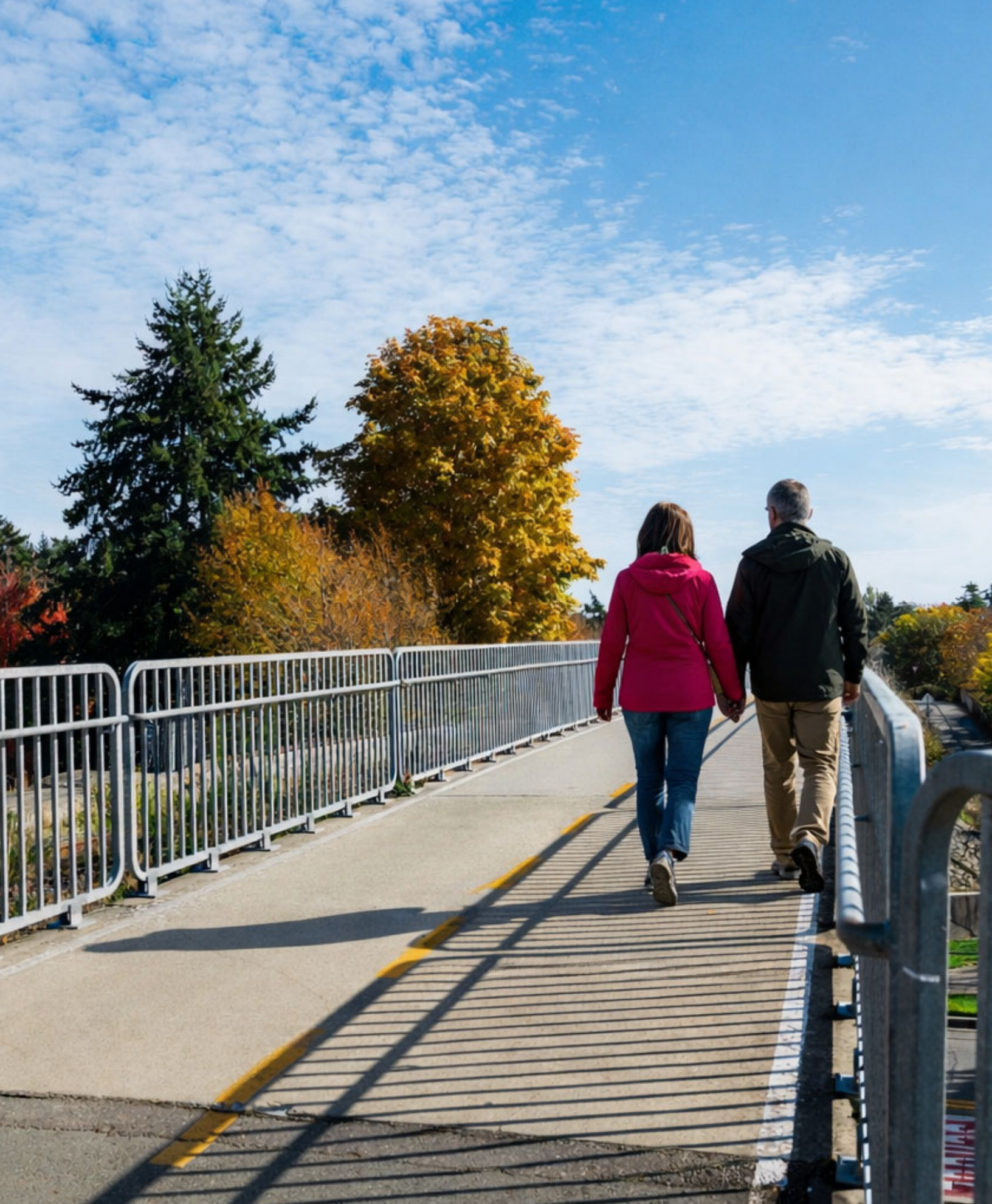
E&N Rail Trail Overpass
